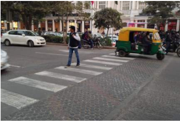
Raised pedestrian crossing
